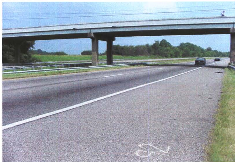
Across Top of Deck
