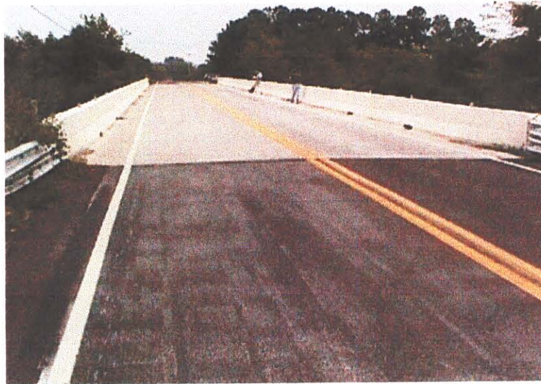
ACROSS TOP OF DECK, NEW DECK & PARAPETS
