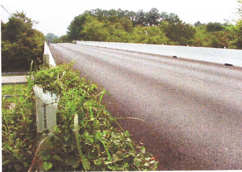
ACROSS TOP OF DECK
